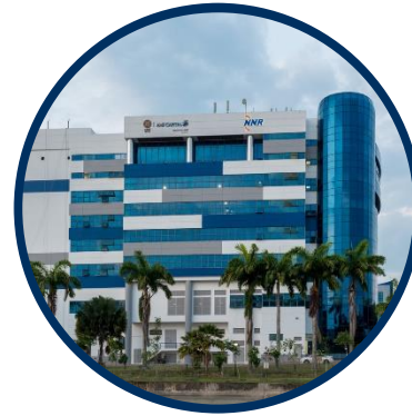
10 Changi South Lane
