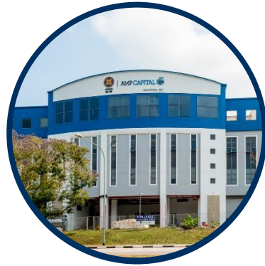
11 Changi South St 3
